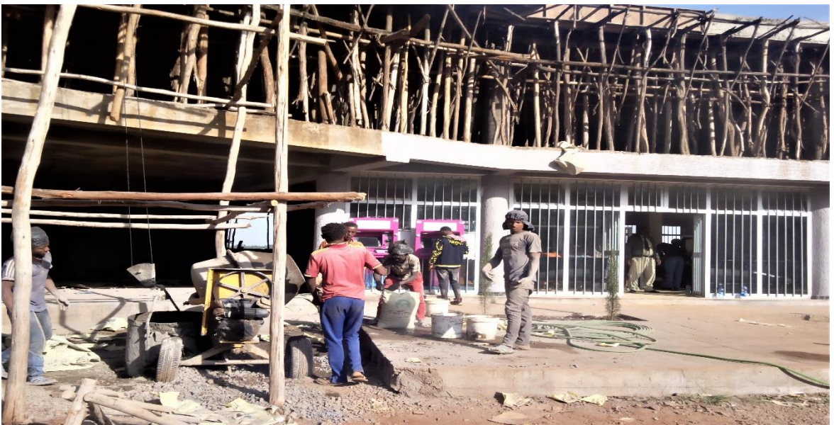
c) Noise and vibration generation from construction site in Wolaita Sodo
