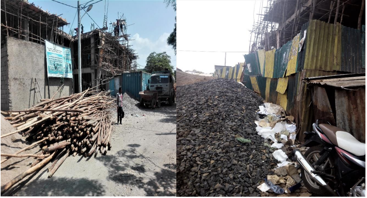
Construction materials and vehicles on the road
