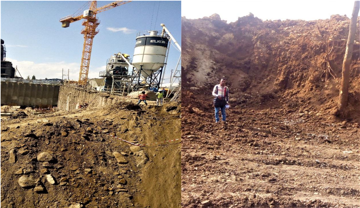
Deep excavation on construction sites
