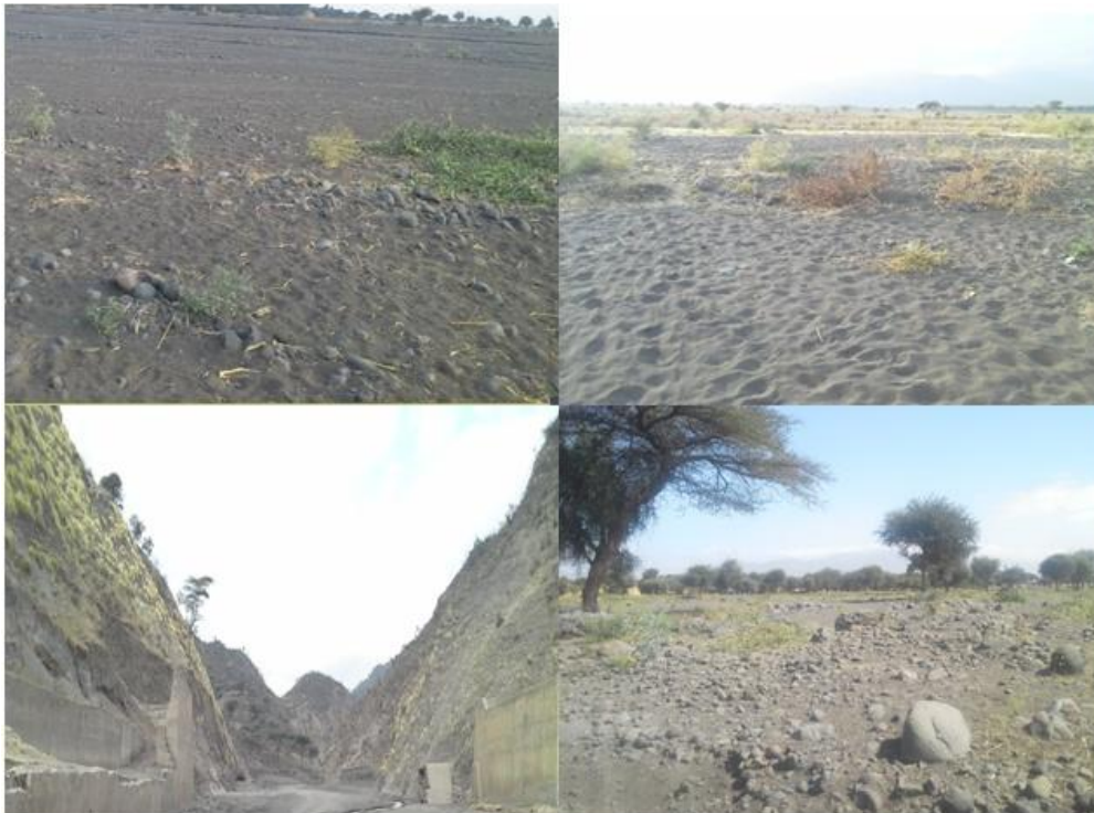
Figure 5 Appendix 2: Diversion Headwork damaged by flood
