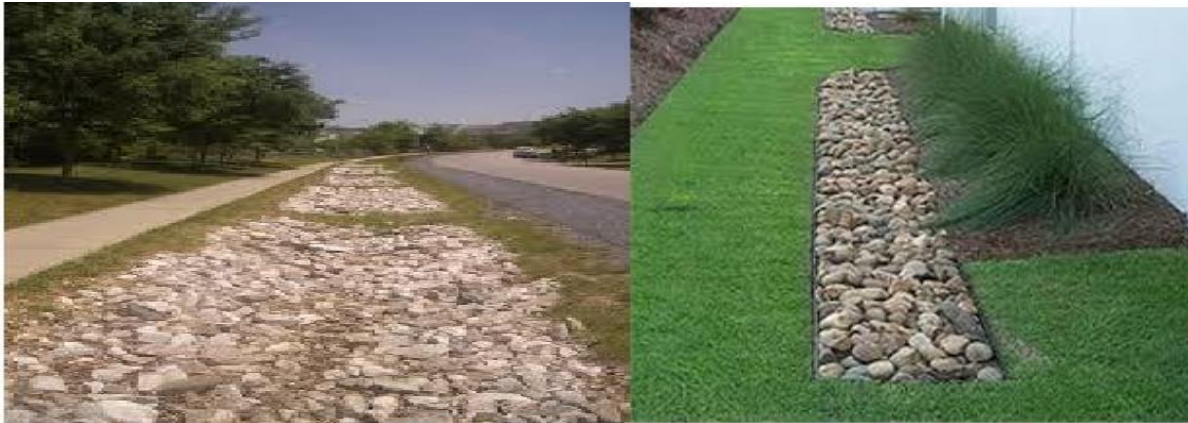
Figure 2: View of infiltration trench structural (EPA, 2015)
