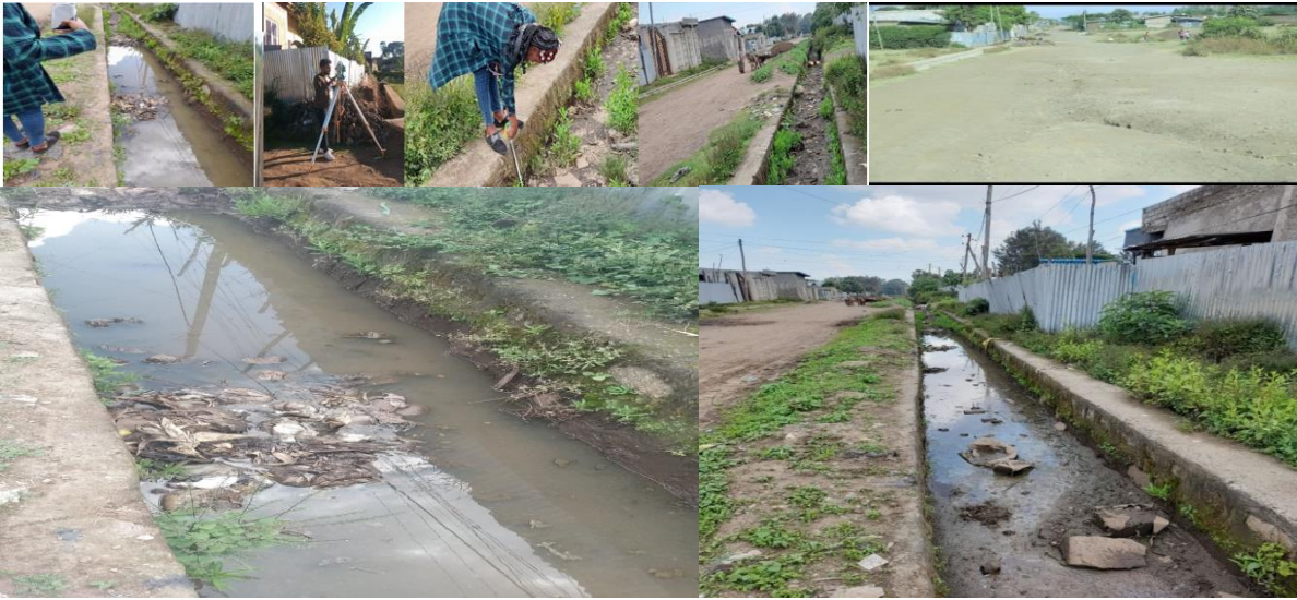
Figure 1: Liquid wastes in to storm drainage (site visiting time)
