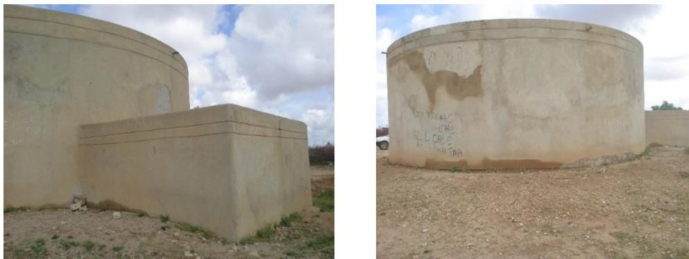
Figure 3-2: Current Status of the existing 350m 3 reservoir
