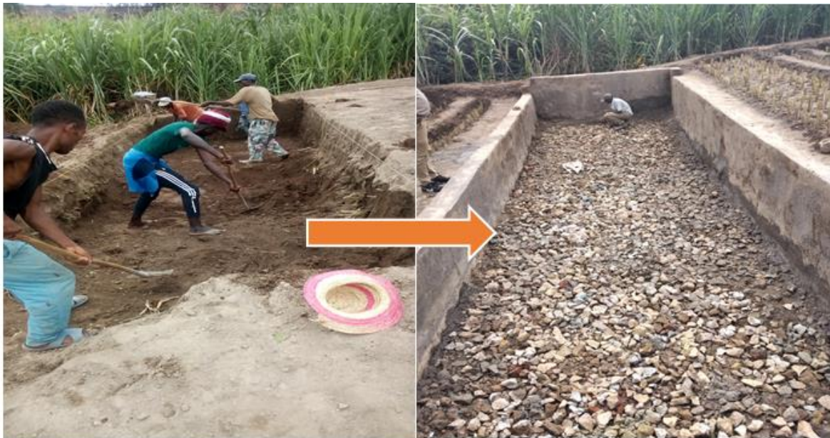
a. During excavation
