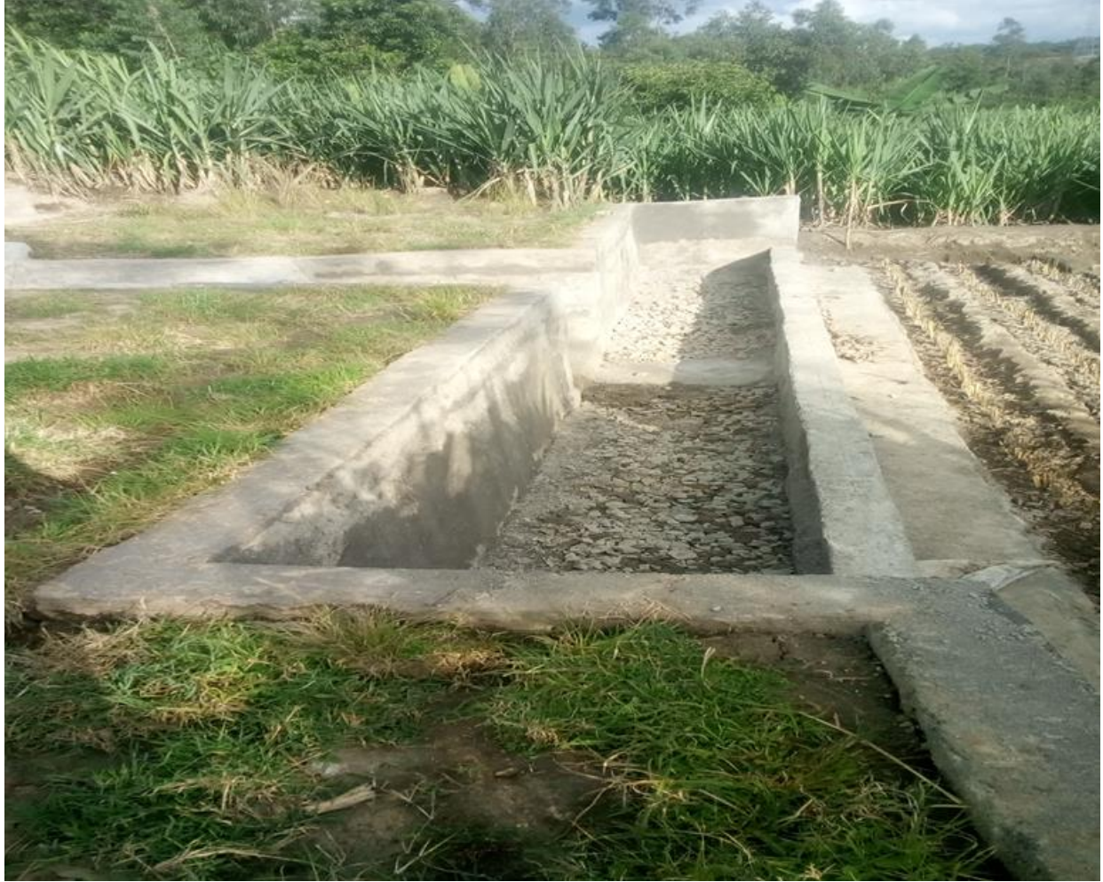
Figure 4.4 Filtration Channel
