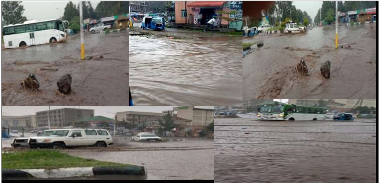
Figure 4. 1: Overtopping due to insufficient carrying capacity hydraulic structure
