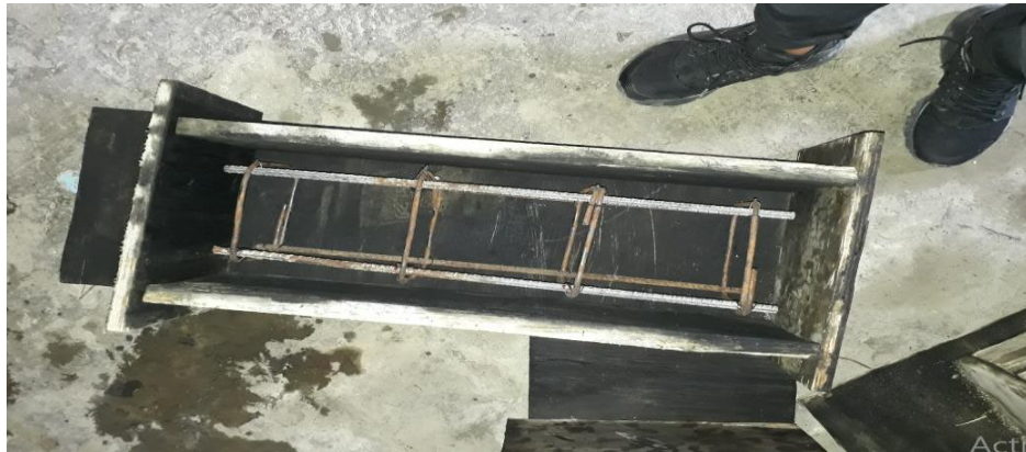
Figure 3.14. Form work and Bar for beams
