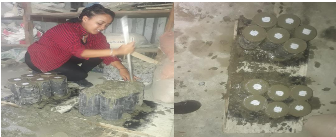
Figure 3.13. Casting of cylinders for tensile strength test
