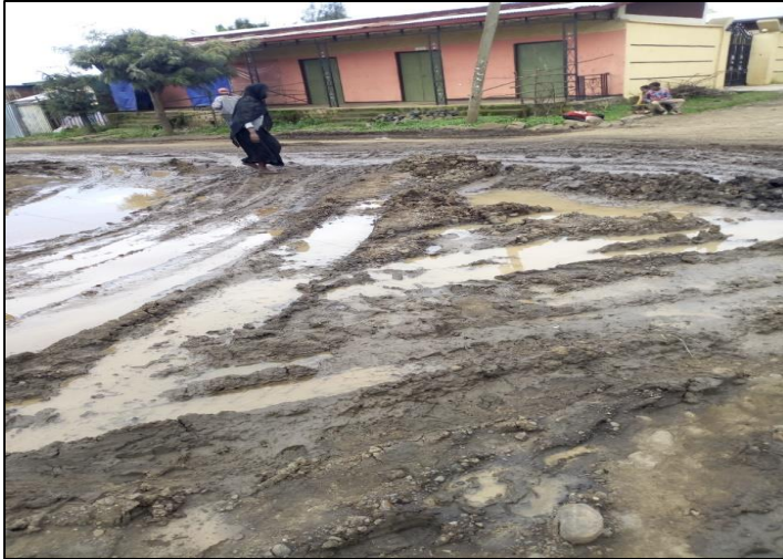
Figure 4.1: Lack of drainage system
