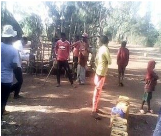
Shamba kebele hand dug well
