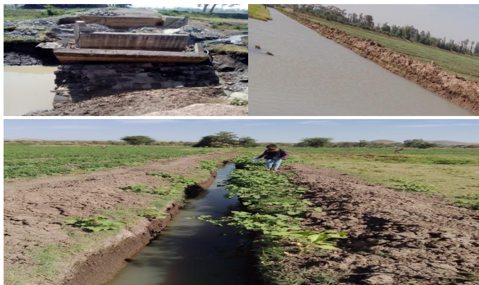
Figure 3. 3: Awash Melkasa irrigation scheme
