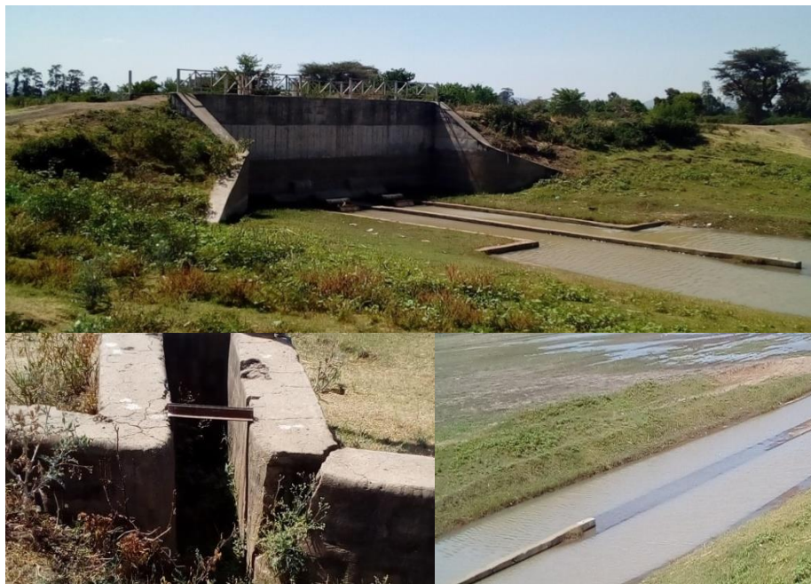
Figure 3. 4: Waqemiya Tiyo irrigation scheme
