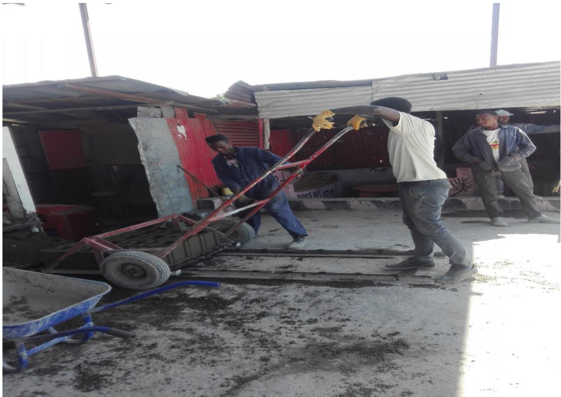
Photo 8. Transportation of extruded green blocks
