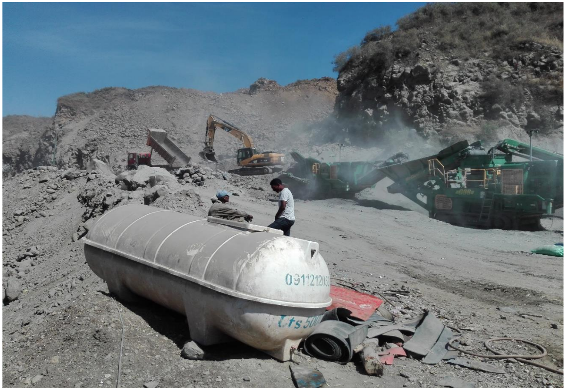
Figure 3.2 Crusher dust produced from crusher site arranged closer to quarry area (Observation around Akaki-Kality sub city)
