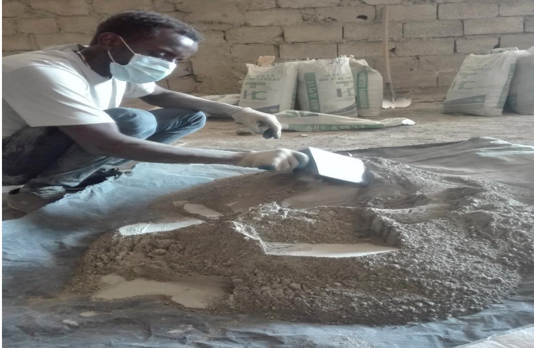
Photo 3. Blending the crusher dust with cement
