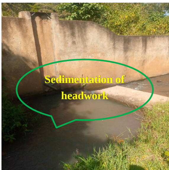
Figure 12:-Photos of damaged structures of Rasa diversion headwork (Source: Author,2024)
