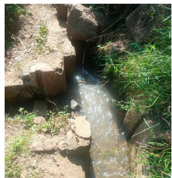
Figure 12:-Photos of damaged structures of Rasa diversion headwork (Source: Author,2024)
