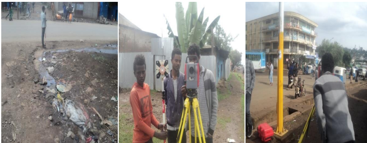
Figure 3.20: surveying the elevation and location junctions by using Theodolite
