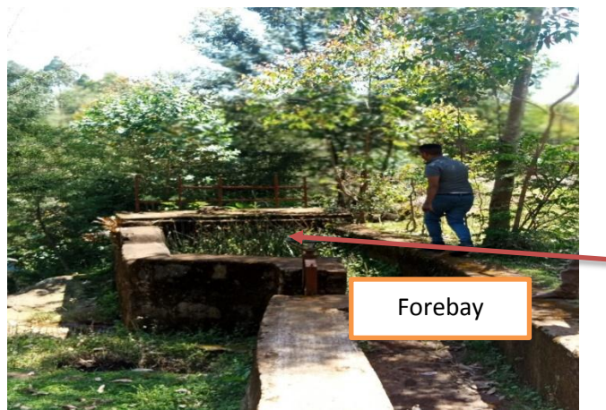
Fig 4.2 Forebay Structure
