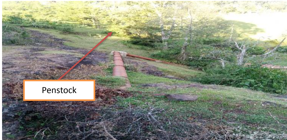
Fig 4.3 Current Condition of Penstock
