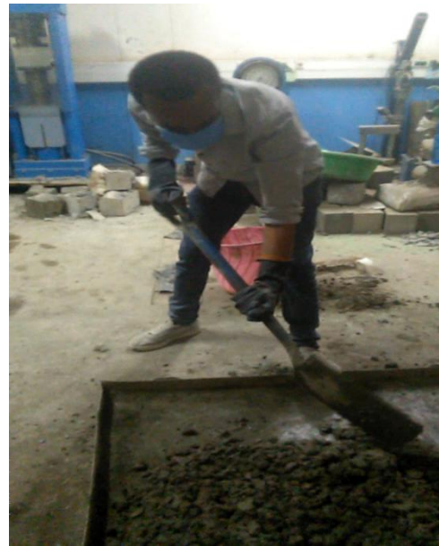
Figure F.10 Hand mixing of fresh concrete
