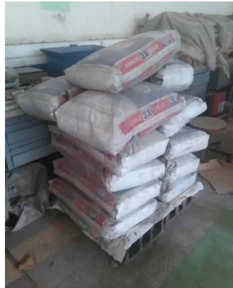
Figure F.8 Cement storage
