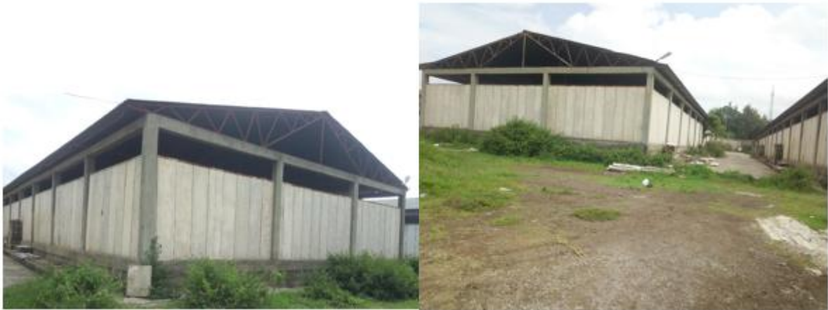
Figure 4.11 Factory store constructed using Agrostone panel
