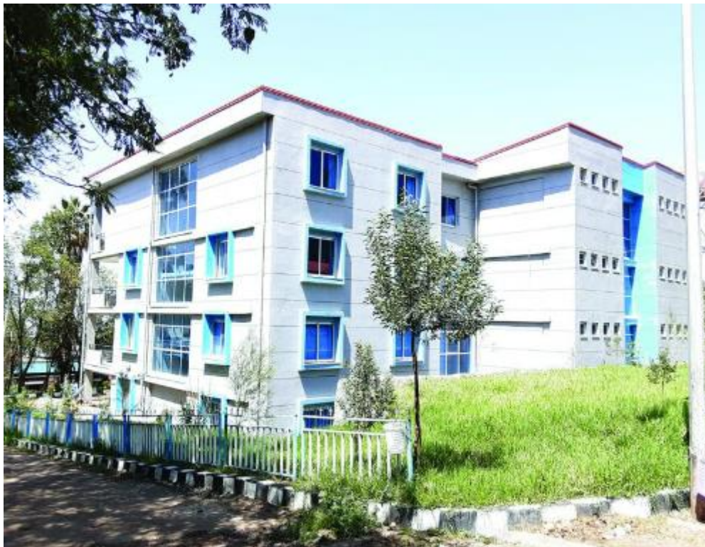
Figure 0.14 Kotebe Metropolitan University 3-story office building constructed using precast concrete by ECWC (photo: AA construction office)
