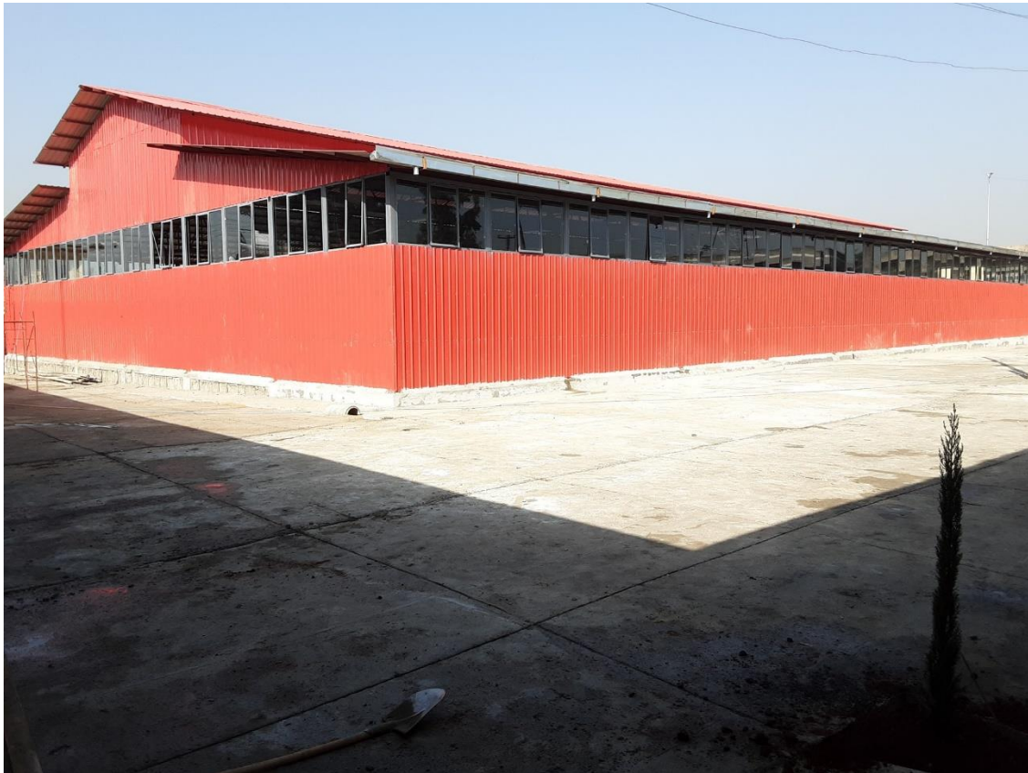
Figure 0.11 Market center constructed using metal sheet and steel frame at Gotera, Addis Ababa (photo: researcher)
