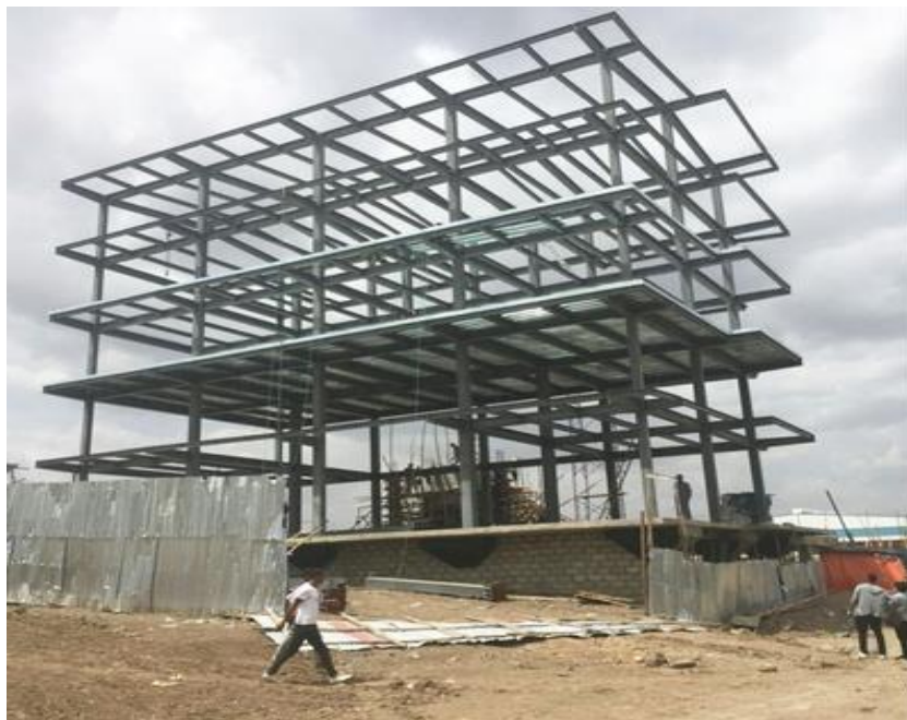
Figure 0.12 Prefab steel frame G+5 office building in Addis Ababa
