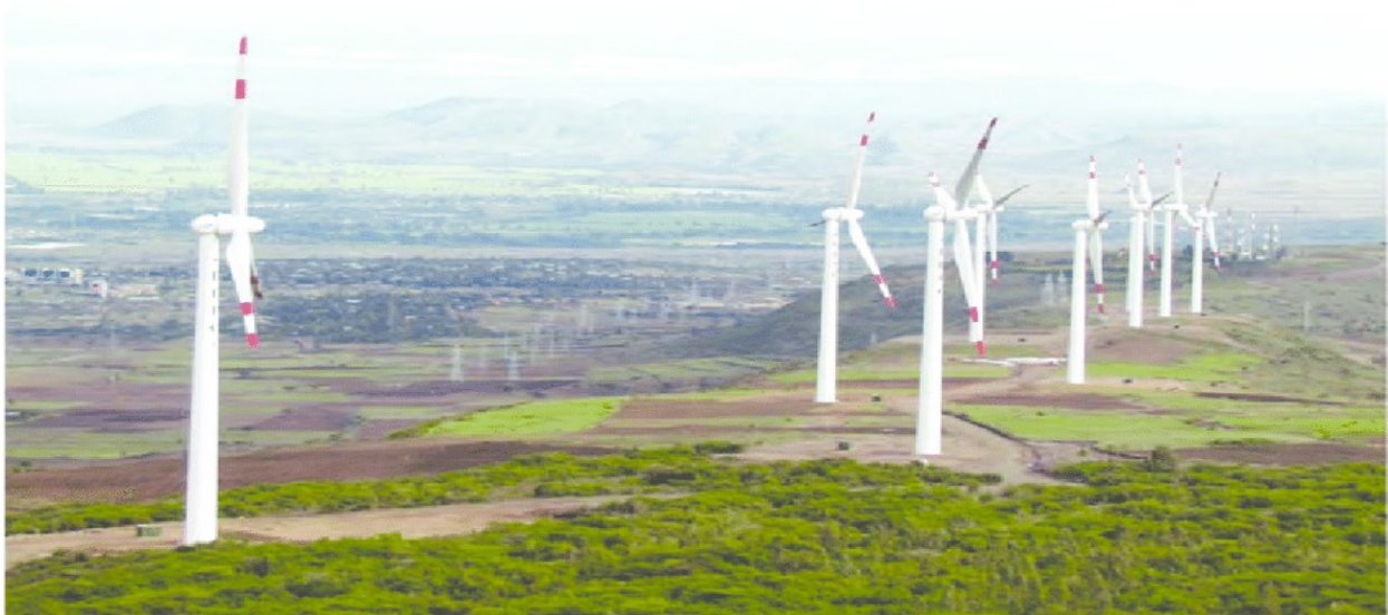
Figure 3.1 Adama I wind farm [58]
