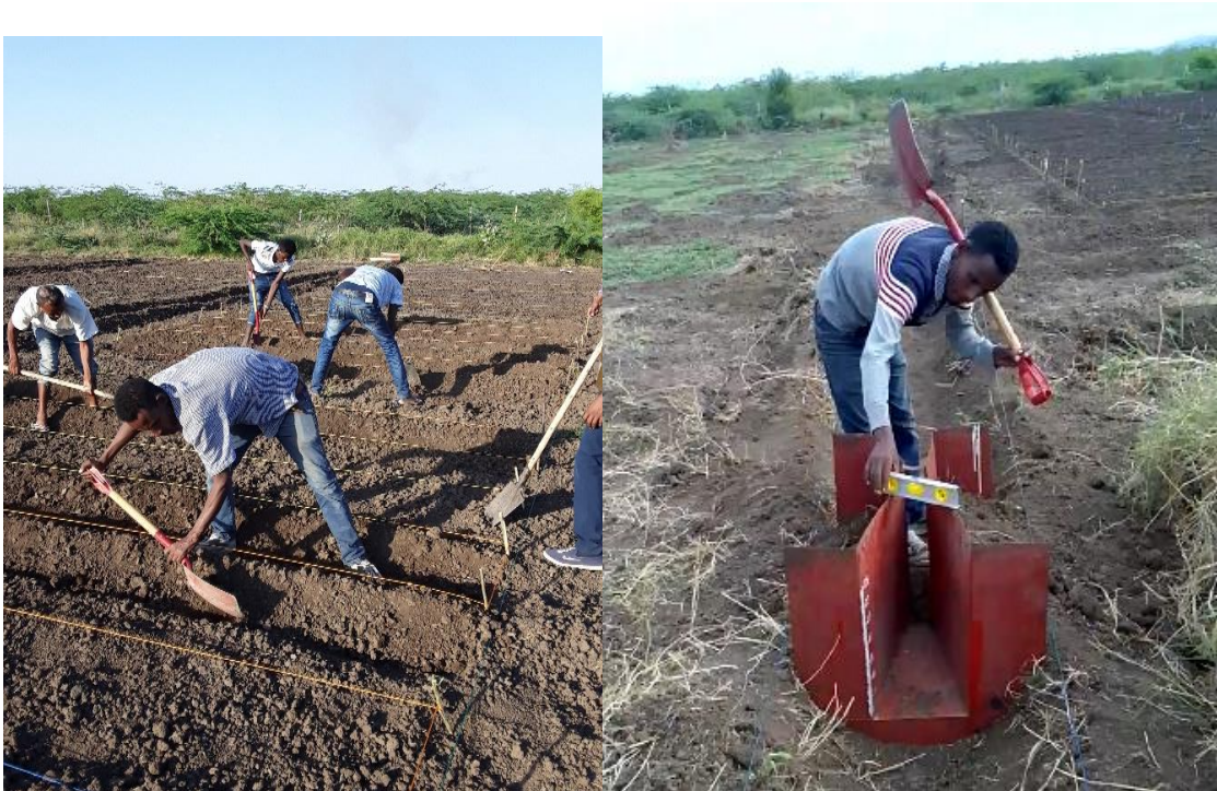
Figure 2. During land preparation and Parshall flume installation in the main canal
