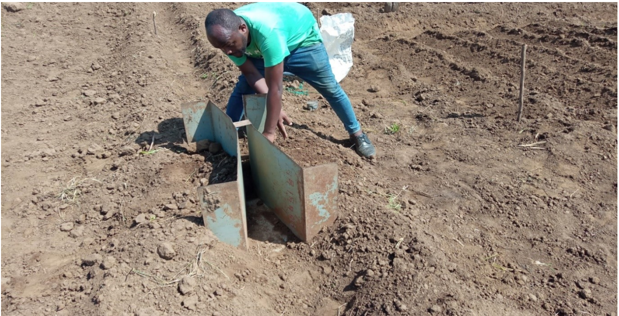
Appendix Figure 10. During soil sampling and parshall flume setting
