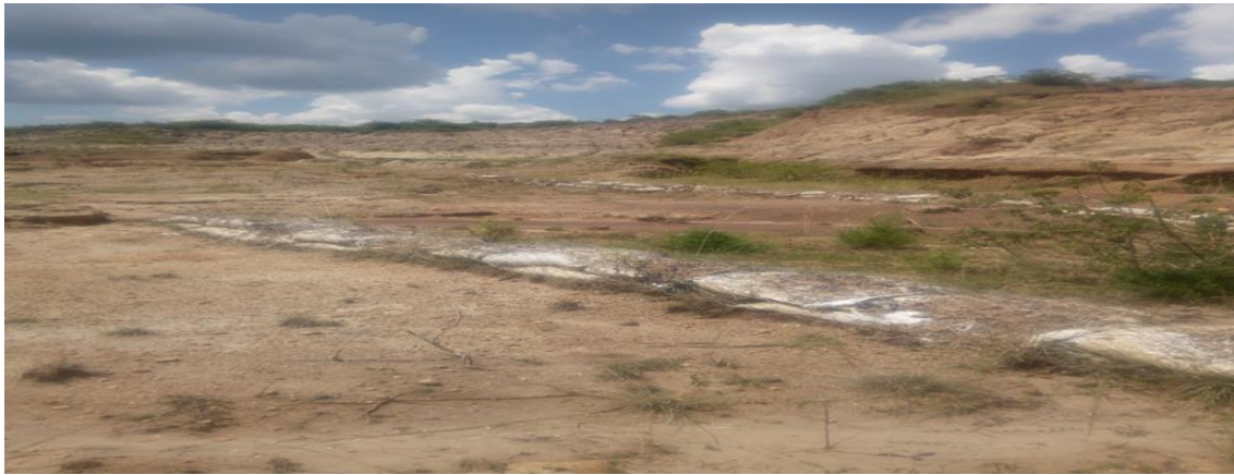
Figure 4. 22 Soil bag check dam
