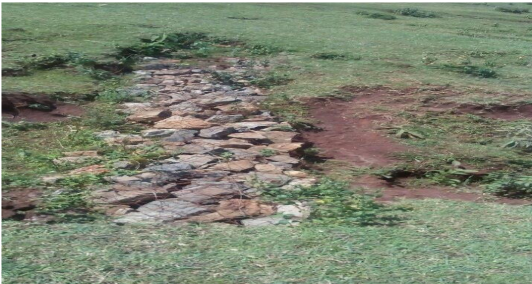
Figure 4. 21 Stone check dam on land affected by soil erosion
