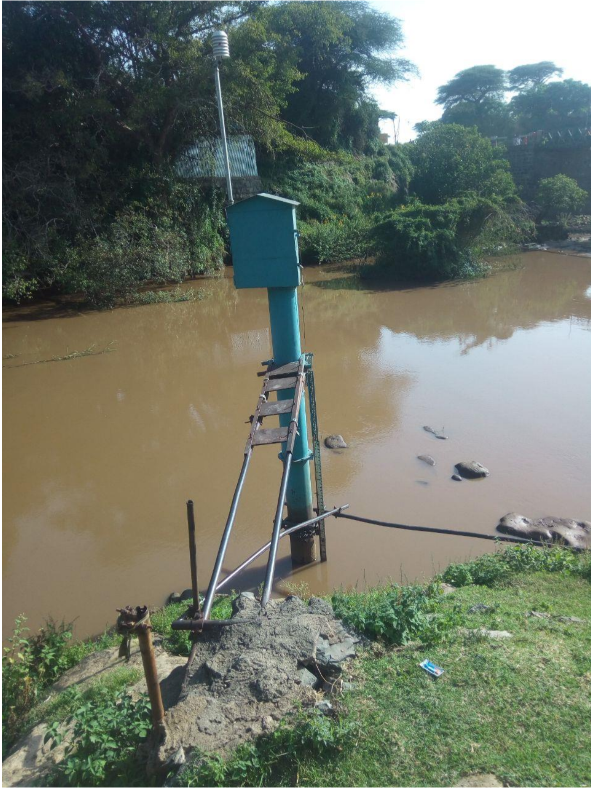
Appendix E; Figure 1:Katar river gauging station at Abura
