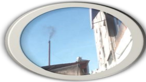
Figure H: A substandard incinerator burns
