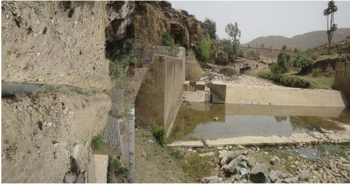
Figure 3. 7: Tsilwe diversion weir structure
