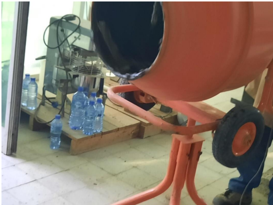
Figure AN. E-12: Concrete mixing
