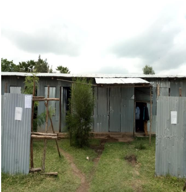
c) Offices used by contractor & consultant in Hawassa project
