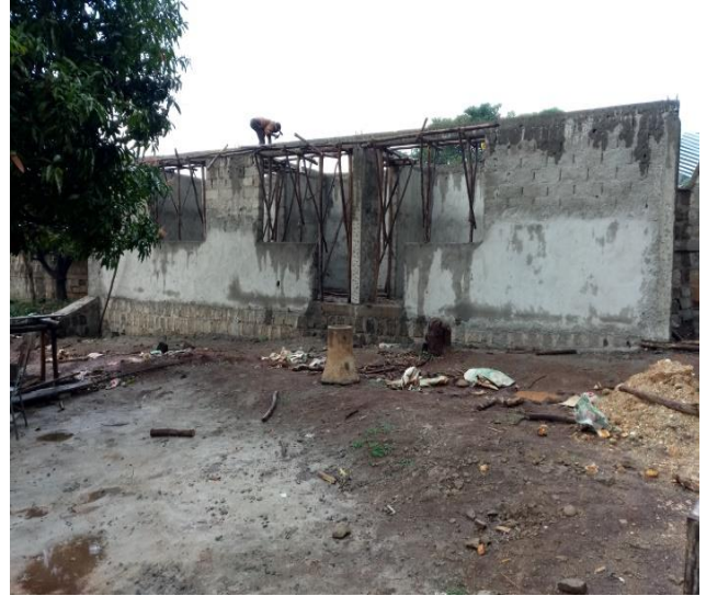
b) Office construction for the consultant in Arba Minch project
