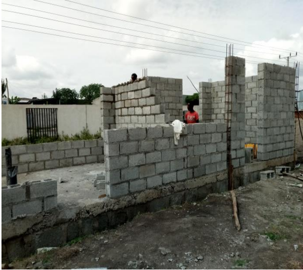
a) Office construction for the consultant in Hawassa project
