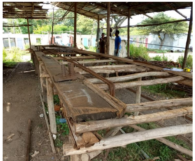
Rebar Storage and Fabrication Yard
