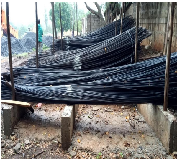
Rebar Storage and Fabrication Yard
