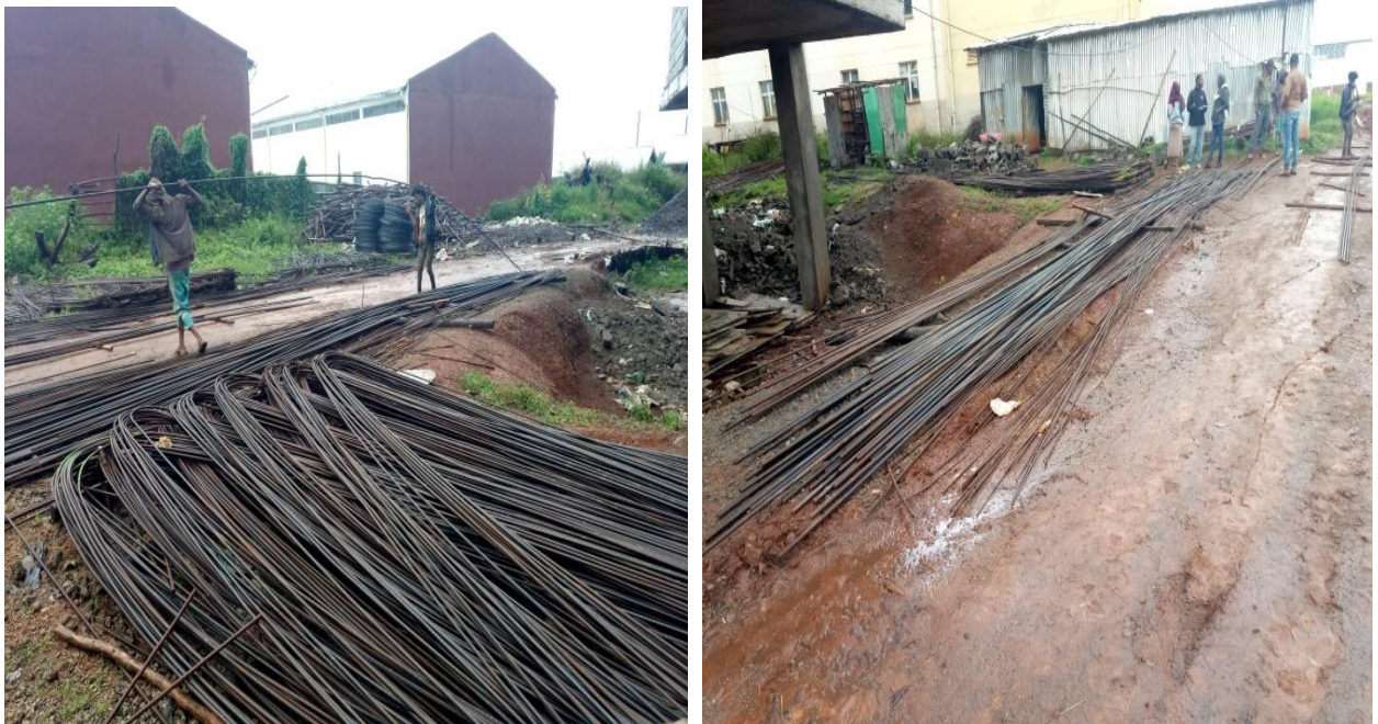
a) Rebar on bare ground in Wollayta Sodo project
