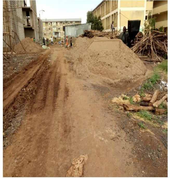
b) Fine aggregate handling in Arba Minch project
