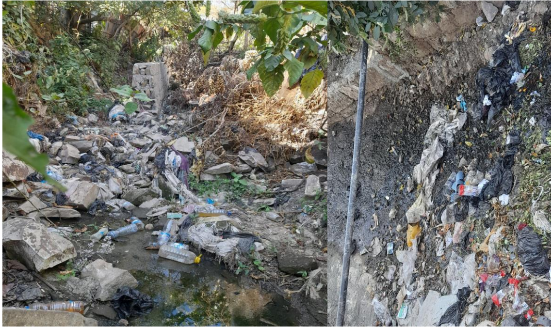
Figure 9 :Solid Wastes Inside Drainage Systems(site visiting time)
