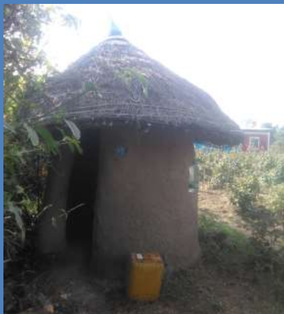
Photo 1: shows the sample photo current HH latrine with Handwashing, 1 st Choroko kebele, Hasan Koricho House
