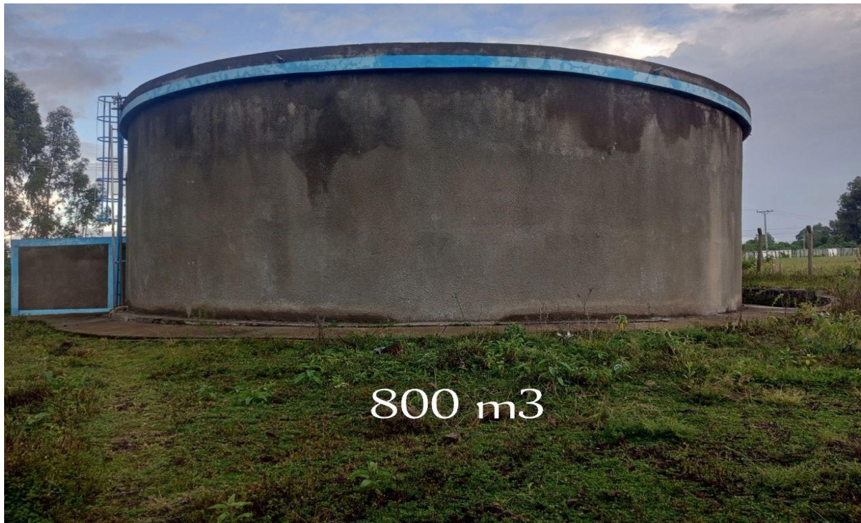
Figure 3 2: The existing 800m 3 reservoir in the Town
