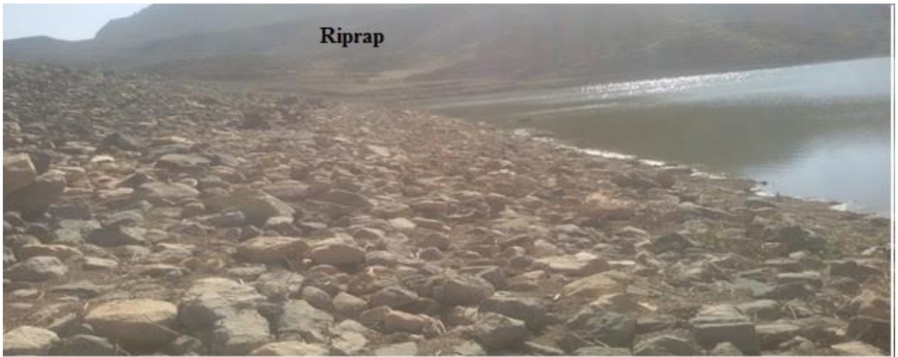
Figure 3.9: photo of riprap zone taken from the site
