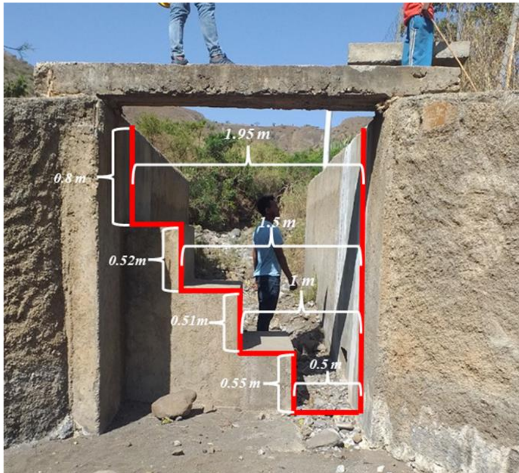
Figure 3-3 Hydrologic monitoring weir (Agewmariam WS)
