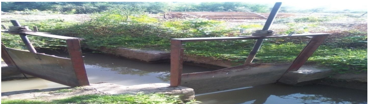
Figure 4: functional division box with gates
