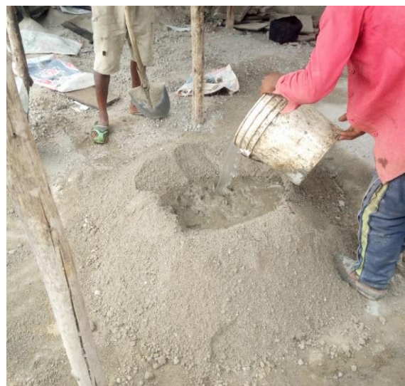
The crushed waste glass mixing for 10%, 20%, and 30% replacements
