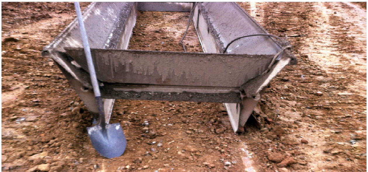
Figure 12: Filter material spreader box
