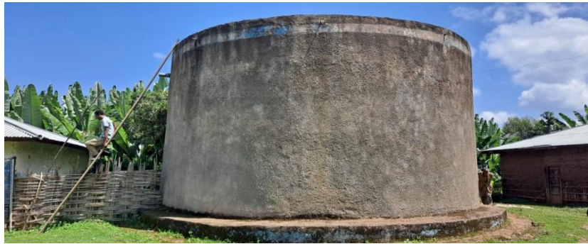
Figure 4.4: Existing service reservoir (Source: field observation, April 2023)
