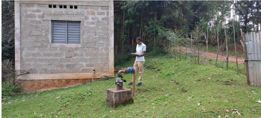
Figure 4.6: Existing well, pump and generator
