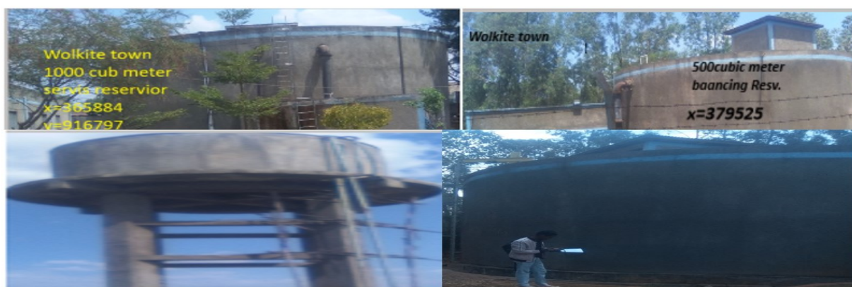
Figure.3.4. Wolkite town Water Reservoir
