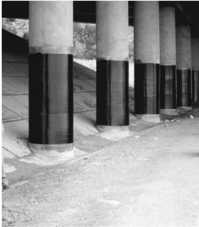
Figure 9 FRP warps being installed on a highway column
