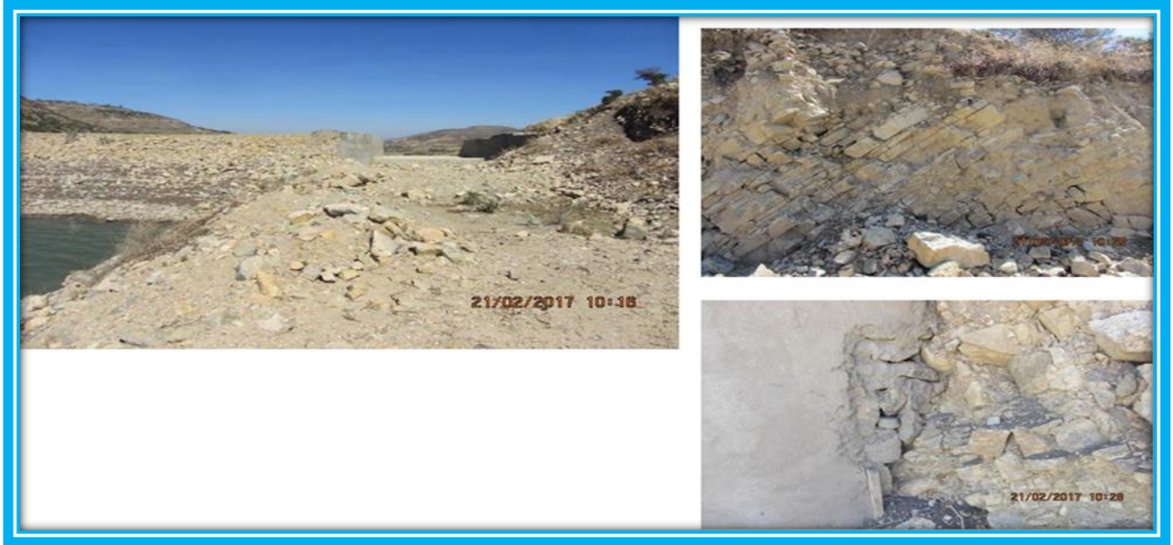
Figure 4.2: Grindeho earth fill dam geotechnical condition and Construction Quality.
