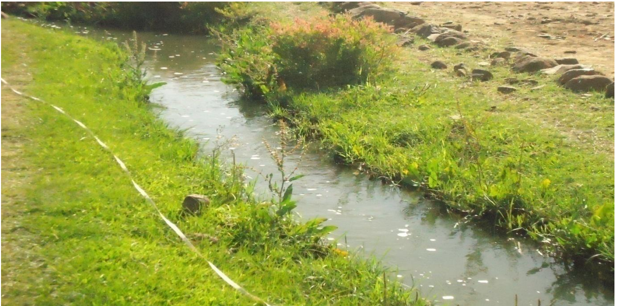
Appendix Figure 4: Unlined secondary canal
