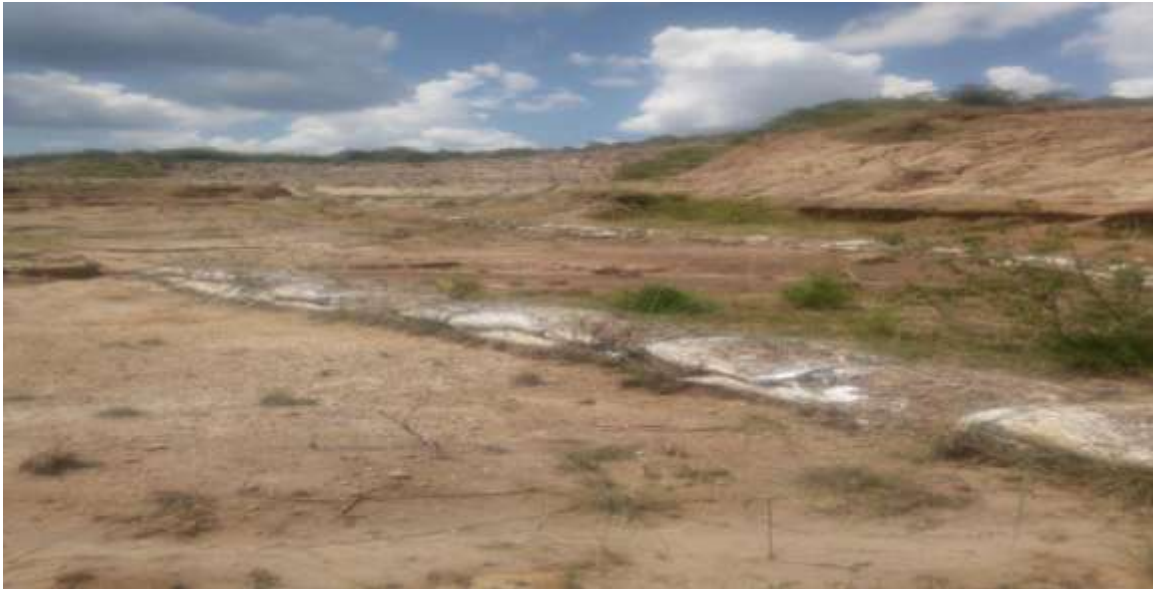
Figure 4 Soil bag check dam
