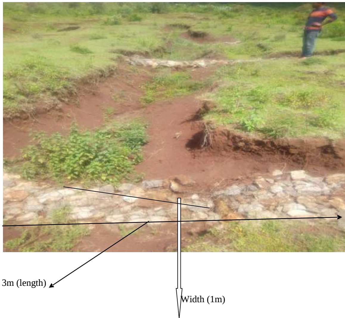
Figure 3 Stone check dam on land affected by soil erosion
