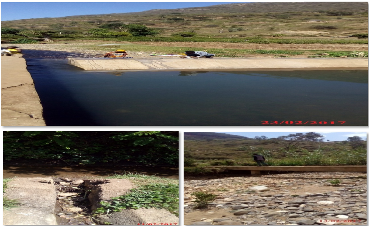
Figure 4.2: Adano scheme head work and current condition of physical structures.
