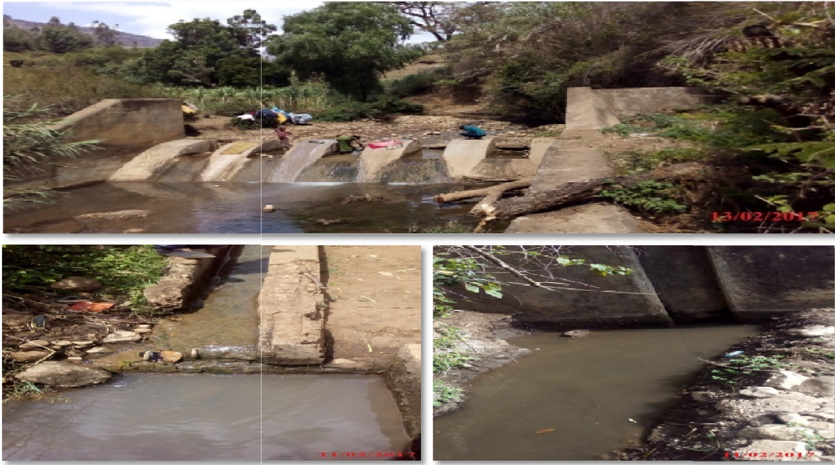
Figure 4.1: Mojo Asha scheme head work and current condition of physical structures.
