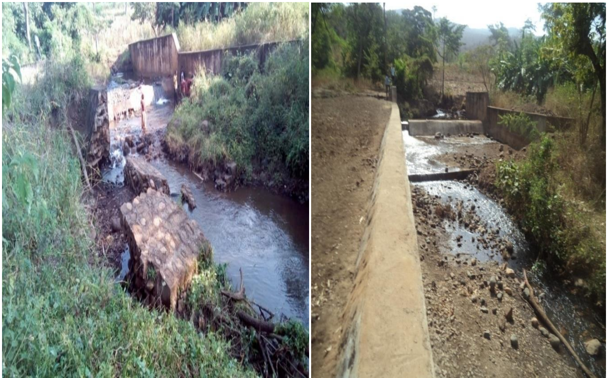
Figure 4. Maintaining and repairing of head work parts of Sanko irrigation scheme
