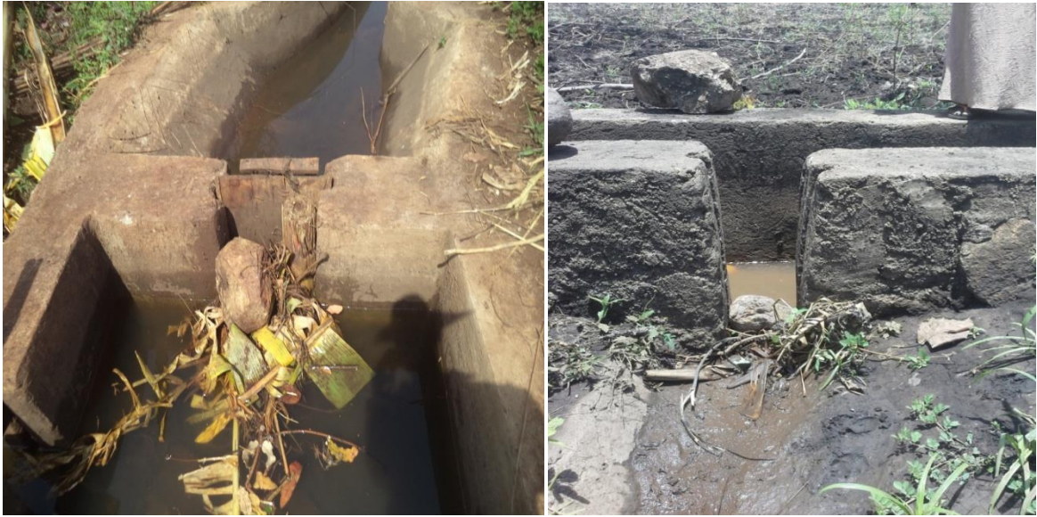
Figure 5. Using earthen materials and stones for opening and closing diversion gates
