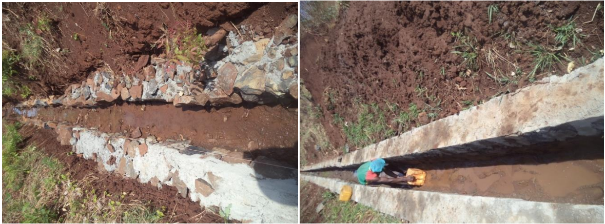
Figure 10. Additional construction of irrigation canal as extension
