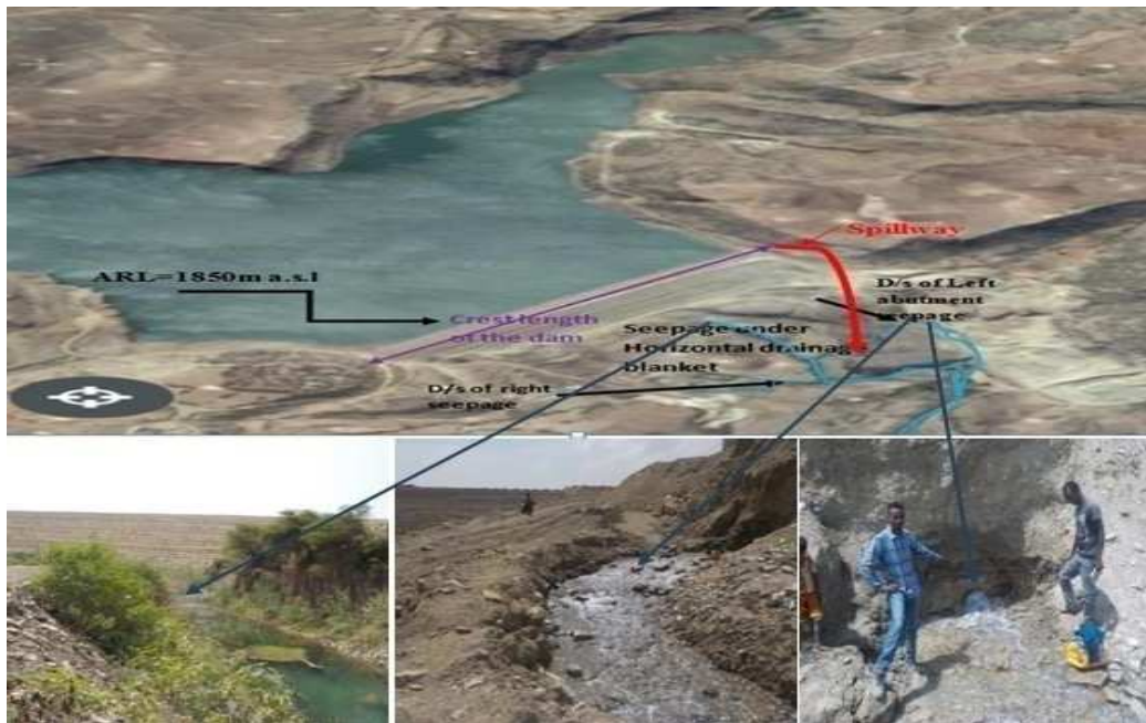
Appendix Figure D: The existing seepage at different location area on the downstream of the dam.
