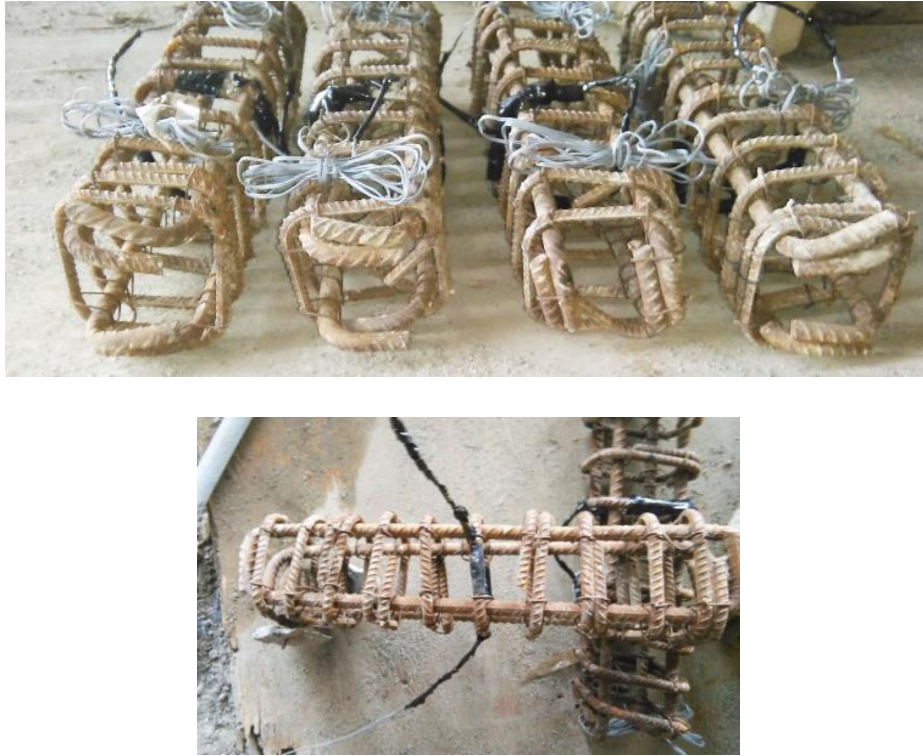
Figure 3. 9 Strain gauges fixed in reinforcement (middle ties)
