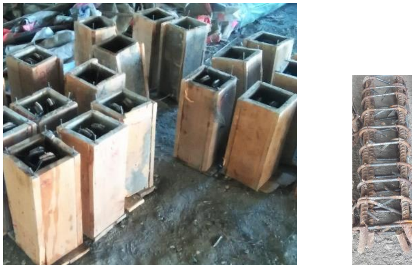
Figure 3. 6 Formwork and Reinforcement cages
