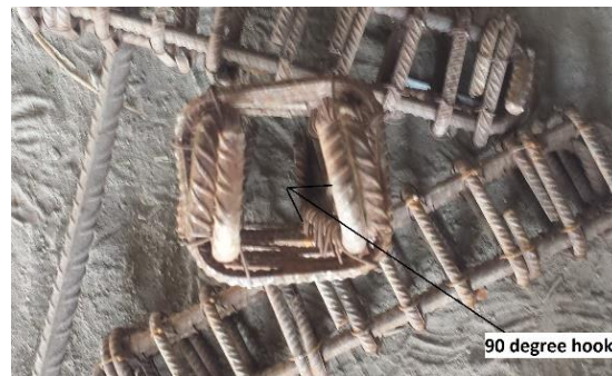
Figure 3. 7 Reinforcement cages and Schematic drawing of reinforcement
