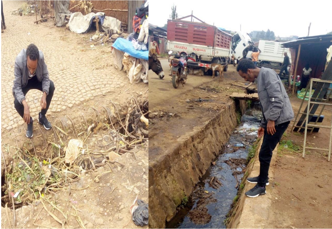
Figure 4. 16 Dumping of solid and liquid wastes in to storm water drainages
