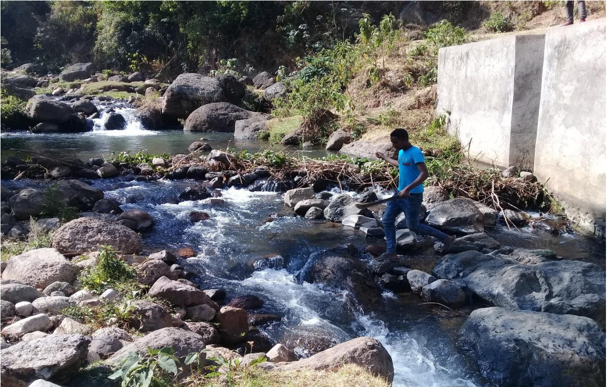
Appendix Figure 2. Werka Irrigation Scheme weir and reservoir
