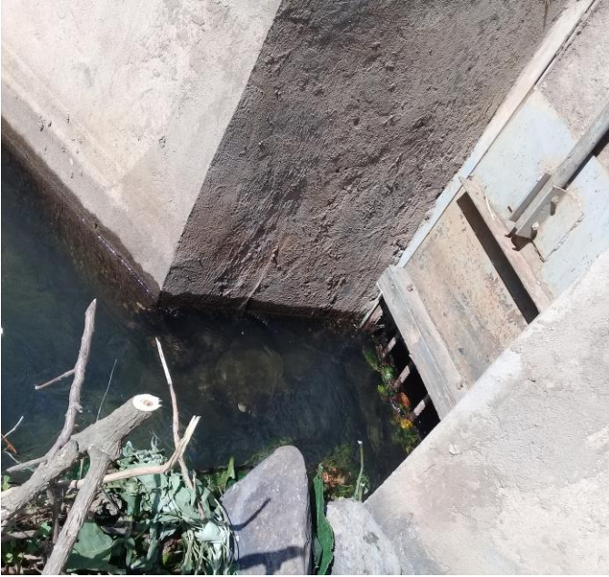
Appendix Figure 8. Nonfunctioning metal sheet gets at Wosha and Werka Irrigation Schemes offtake canals
