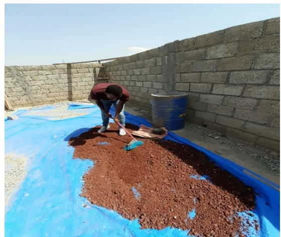
Figure 3.3B) Air drying lateritic gravel
