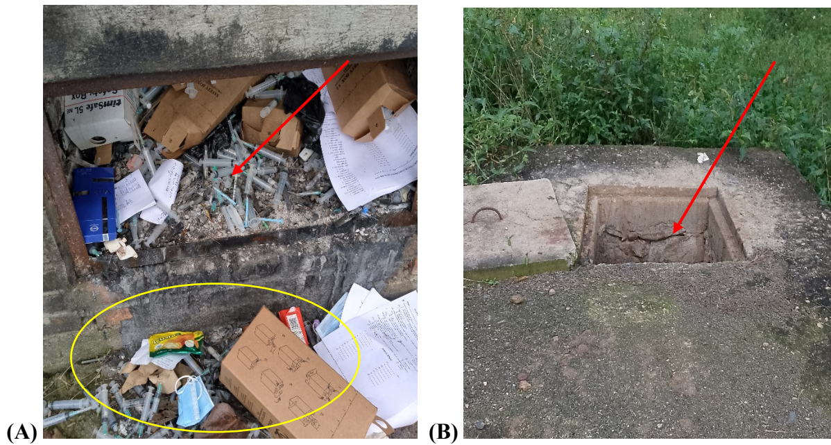
Figure 12: Photo shows, dumping of waste in old brick incinerator (figure A), open and unsecured placenta pit (figure B) in Kelle Primary Hospital, February 2024
