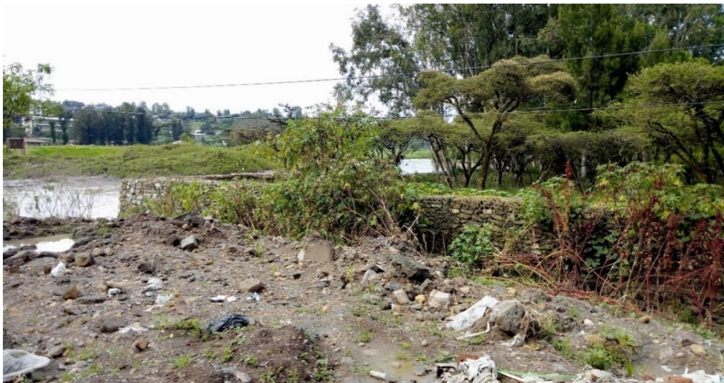
Figure 4.13: Current existing flood protection works (gabion)
