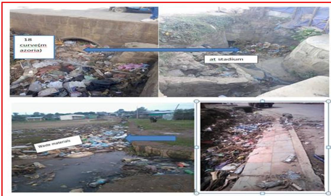
Figure 20: Drainage Nodes are blocked by solid wastes in study area
