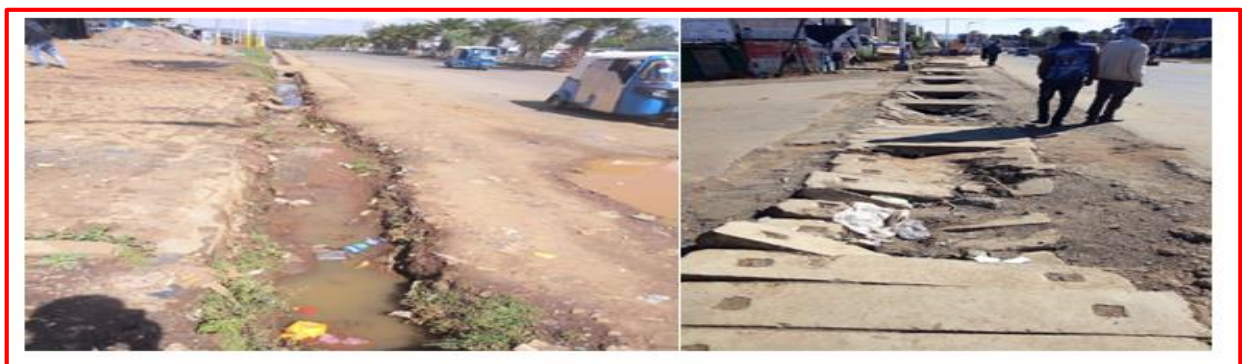
Figure 17: Abutment erosion (left) and cracked slab (right).
