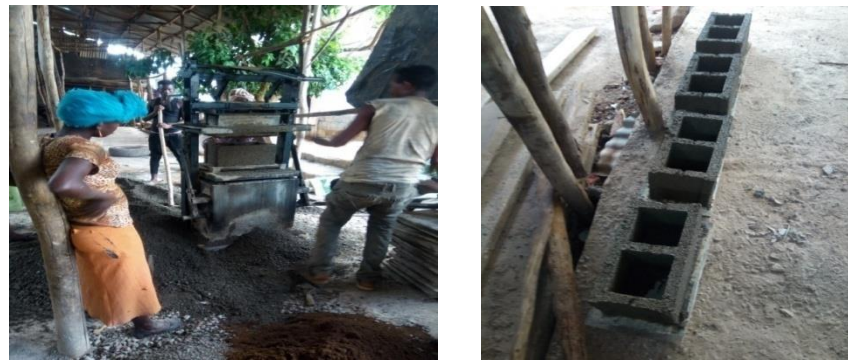
Figure 4.35 - compacting and placing of HCB in Walelign HCB production
