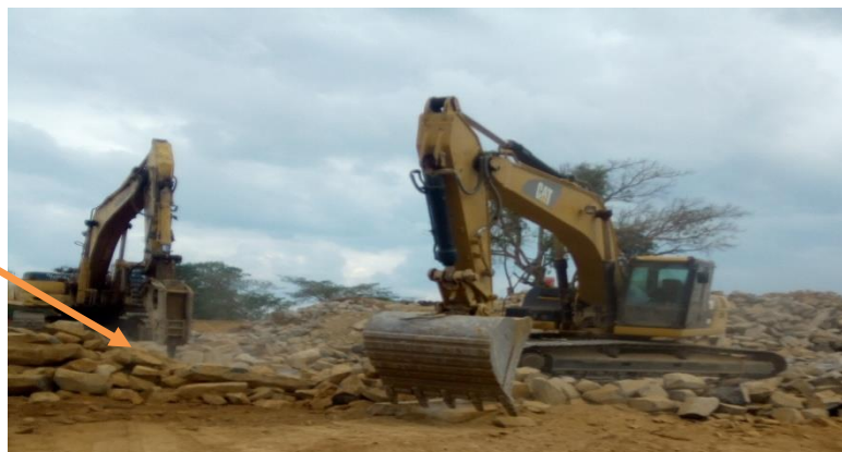
Figure 4.1 Pre-Production Crushing on wenago crushing site
