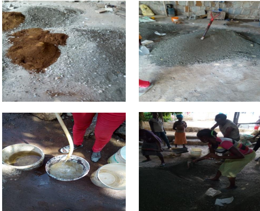
Figure 4.33 - mixing process in Waleign HCB production
