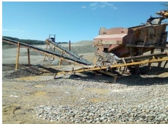
Figure 4.23 Screening in Golla Crushing Site
