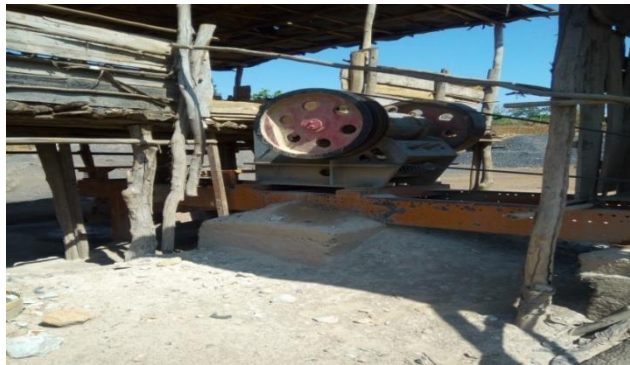
Figure 4.5 Small Crushing Machines on Waleme Crushing Site
