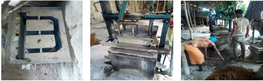
Figure 4.34 - molding of HCB in Walelign HCB production
