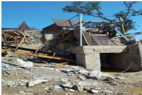
Figure 4.21 Primary Crusher of Golla Crushing Site
